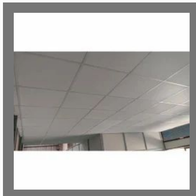
PVC Ceiling Work
