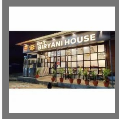
Front Elevation ACP Work
