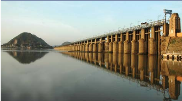
Prakasam Barrage Project Andhra Pradesh
