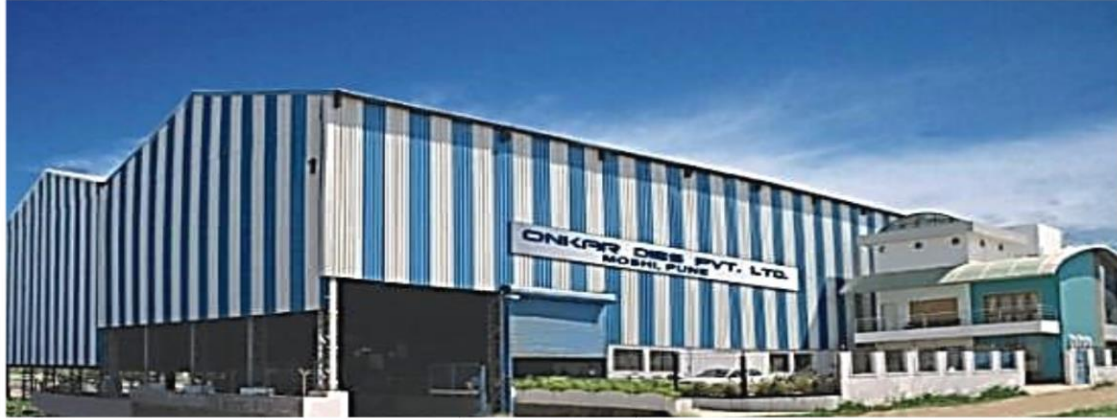
TOOLING BUSINESS UNIT J-140, MIDC BHOSARI, PUNE.
