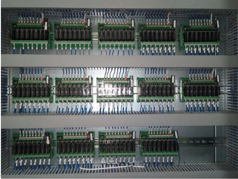
Relay Board Component Plate Wiring Assembly
