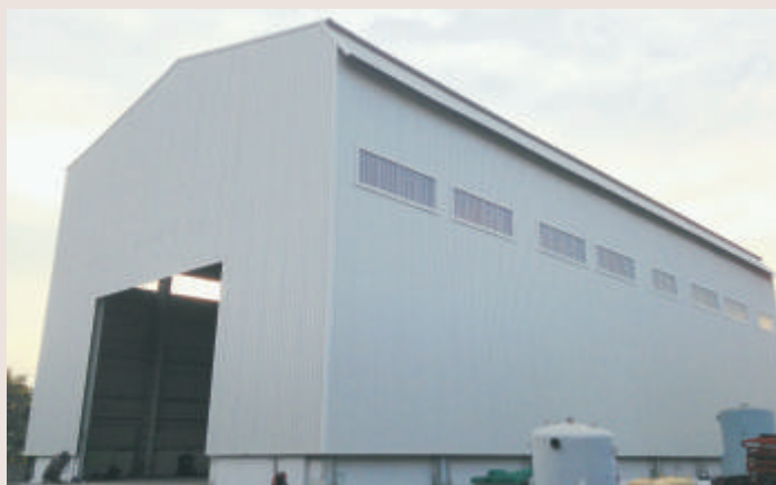
Shop No. 2 - 20 Mts x 45 Mts with 11 Mts Hook Height 15MT Double Girder Cranes - 2 Nos
