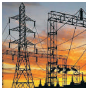
POWER GENERATION & DISTRIBUTION CENTERS
