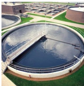
WATER TREATMENT PLANTS
