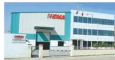
HEMA DRIVELINE & HYDRAULICS PVT LTD Location : Chakan, Pune, Maharashtra Duration : 4 Month Usage : PEB + CIVIL
