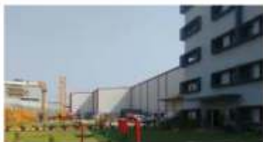
Manitowoc Cranes - Potain India PVT LTD Location : Chakan, pune, Maharashtra Duration : 16 Month Usage : CIVIL + PEB + MEP
