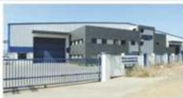
AT & F INDIA FABRICATION PVT LTD Location : Chakan, Pune, Maharashtra Duration : 11 Month Usage : PEB + CIVIL
