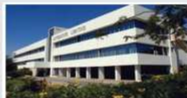
RINDER INDIA PVT. LTD. Location : Chakan, Pune, Maharashtra Duration : 4 Month Usage : PEB + CIVIL
