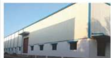
TAIKISHA ENGINEERING INDIA PVT.LTD. Location : Kondhapuri, Pune, Maharashtra Duration : 4 Month Usage : PEB
