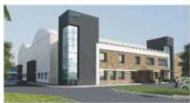
DMW INDIA PVT LTD Location : Chakan, pune, Maharashtra Duration : 6 Month Usage : CIVIL
