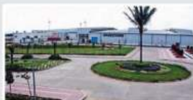
BRIDGESTONE INDIA PVT LTD Location : Chakan, Pune, Maharashtra Duration : 6 Month Usage PEB
