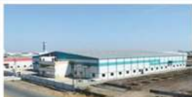
VIGNAHAR STRUCTURE PVT LTD Location : Chakan, Pune, Maharashtra Duration : 12 Month Usage : PEB + CIVIL
