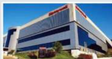
HONEYWELL INDIA PVT LTD Location : Hijewadi, Pune, Maharashtra Duration : 3 Month Usage : PEB + CIVIL
