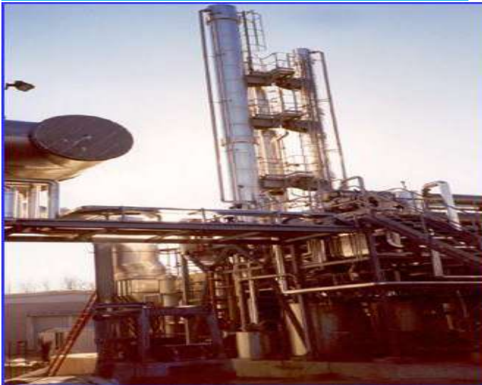
Double effect IPA distillation
