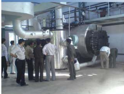
3-PASS FULLY WET BACK
